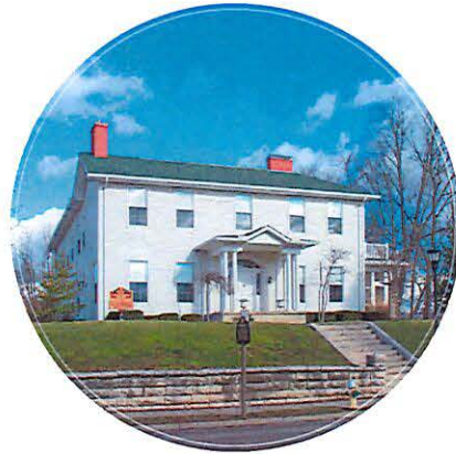
OTHER BUILDINGS Corwin House 210 W. Main Street
