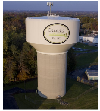
20 Mile Elevated Water Tower
